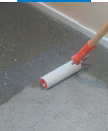
Applying Primer G with a roller
