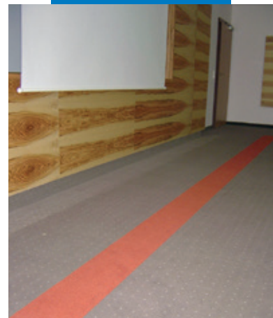
Example of Primer G applied before spreading on Ultraplan Eco and Rollcoll adhesive, used to bond carpet in a hotel room - Villa Hotel Castellani - Austria
